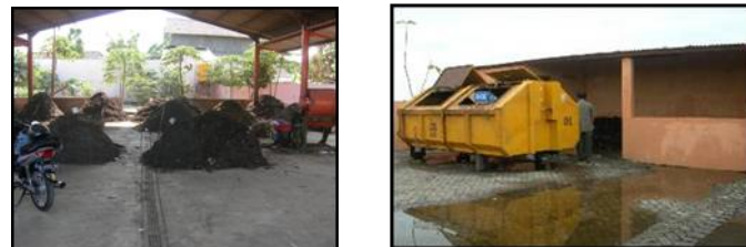
Front-view of composting center at transfer site (Surabaya city & Jombang regency)
